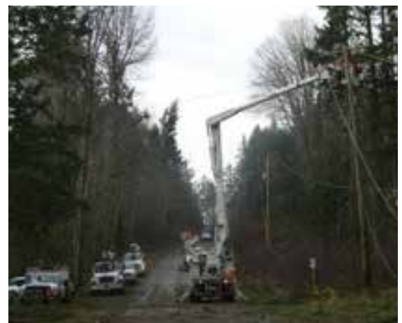
Crews repairing extensive damage in Nanaimo.
